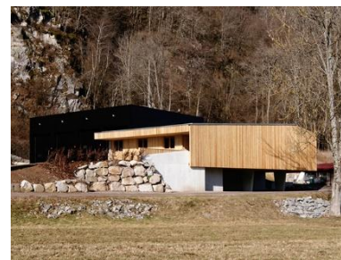
Figure 3. Fire station in reserve "Ballon des Vosges ". France. 2017 [17].
