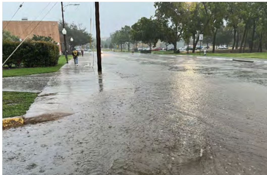
Greek Row flooding corrections – stormwater contained largely in right of way after improvements (Source: UTA)
